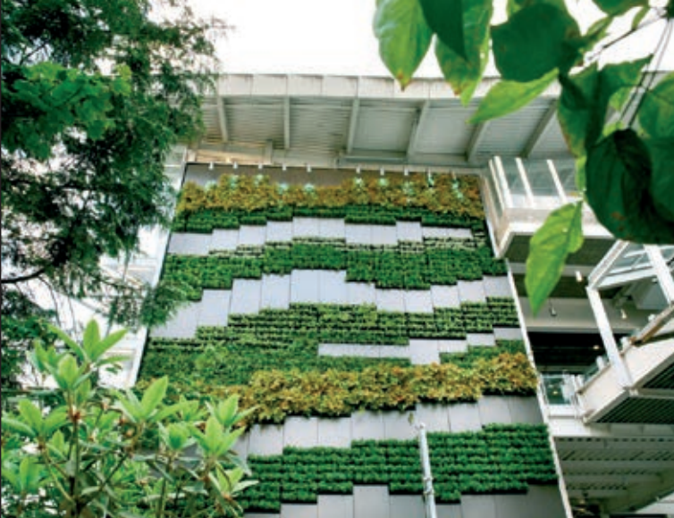
Muro verde: Vancouver Airport Living Wall's, GSKy, Vancouver, Canada.
