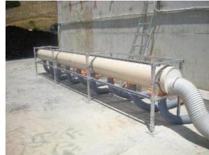
**LA COPERTURA Q-RING™** RIDUCE L'UMIDITÀ E FILTRA L'ARIA PRIMA DELL'EMISSIONE IN ATMOSFERA
